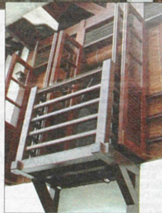
Beauty and function: The walls, windows and floors are made of cengal , a beautiful, durable wood.
