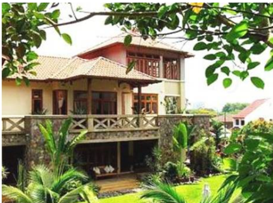
The double-storey structure has lots of wide, wraparound terraces and balconies from which to enjoy the lush greenery surrounding it.
